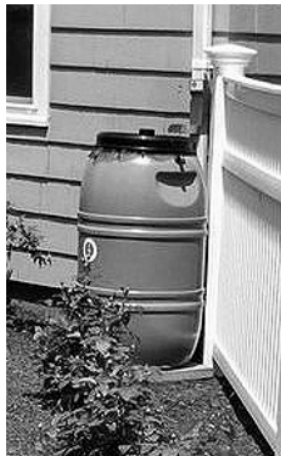
Rain barrels or larger cisterns collect water during storms for later use in gardens, car washing etc.
