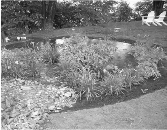
Rain gardens or bioretention systems hold water during storms and release it slowly.
