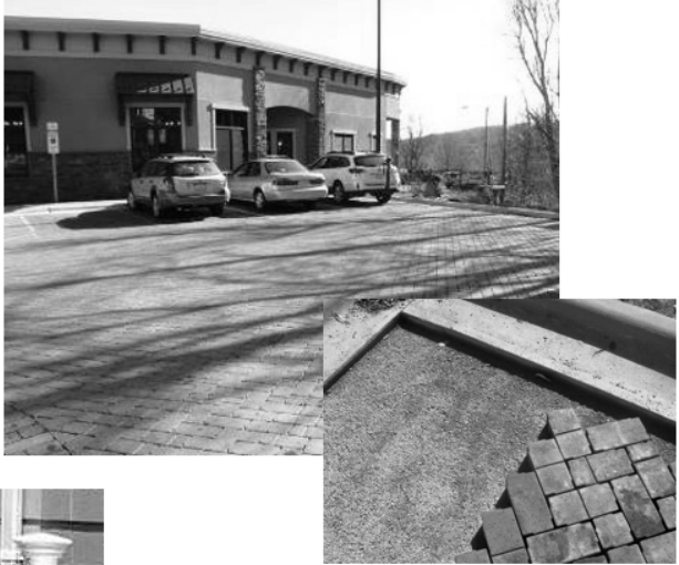
Permeable pavement allows water to soak through it rather than running off of it.
