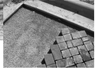
Permeable pavement allows water to soak through it rather than running off of it.
